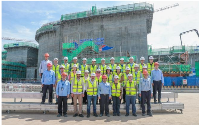
Visit to the SMR Engineering Sites.
